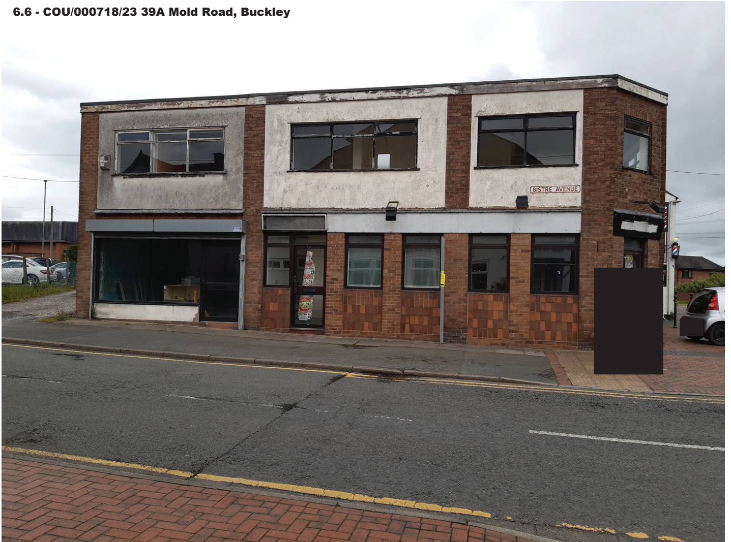
6.6 - COU/000718/23 39A Mold Road, Buckley
