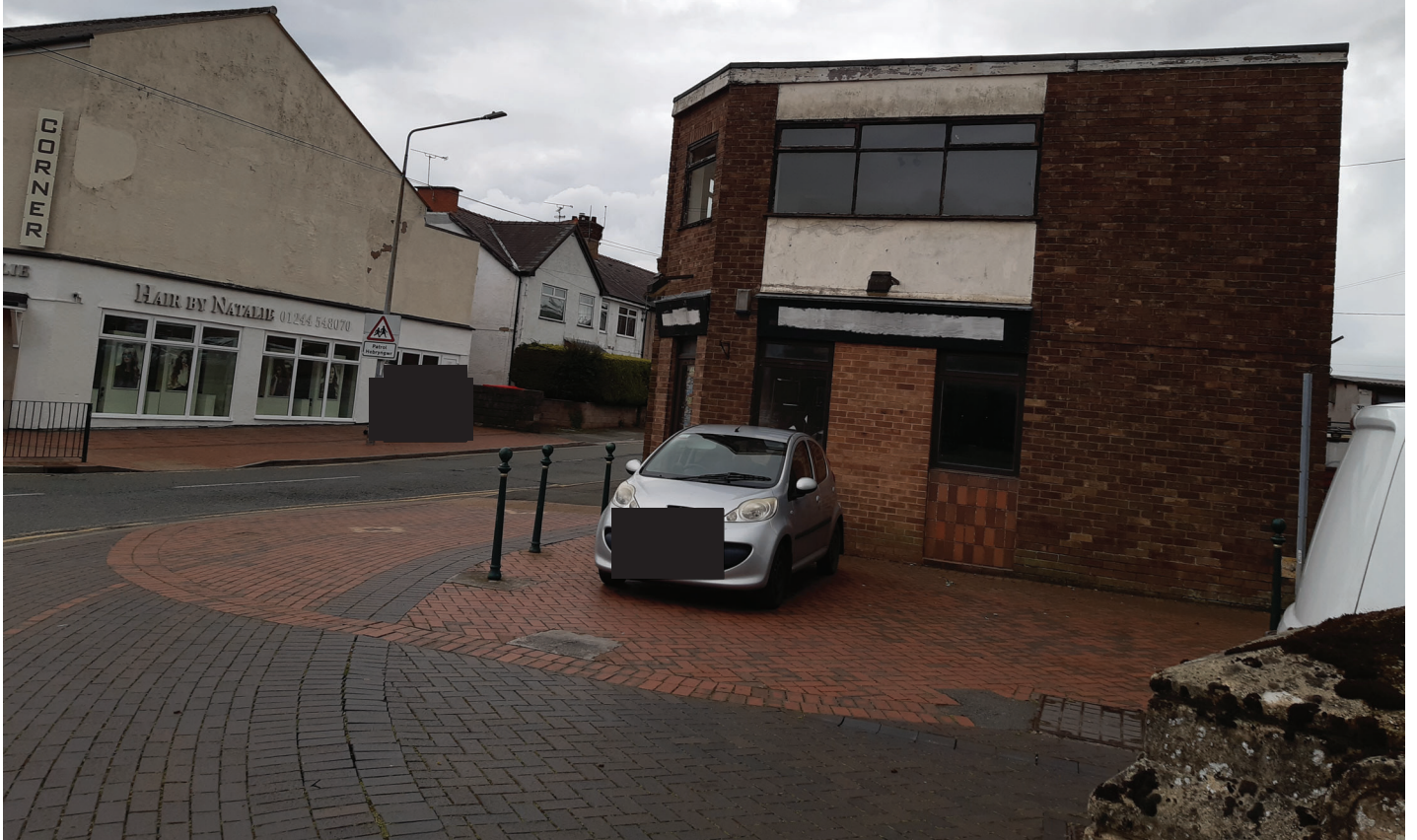
6.6 - COU/000718/23 39A Mold Road, Buckley
